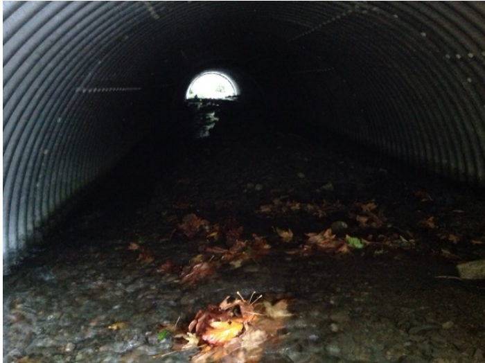
looking through culvert from upstream
